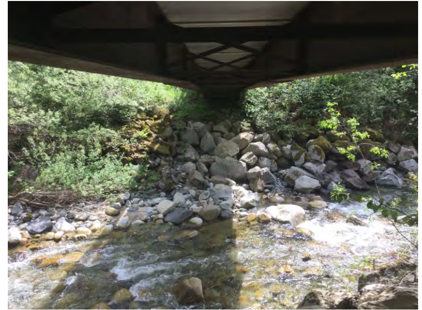
Approach from Left Bank when facing downstream
