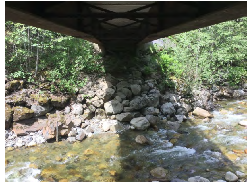
Right Bank Abutment when facing downstream
